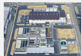
Waste liquid treatment plant
