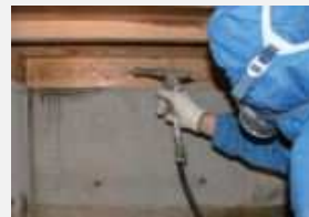
Termite control construction
