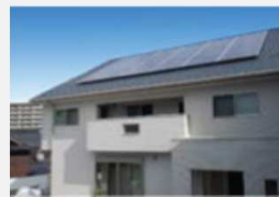
Residential solar power generation system
