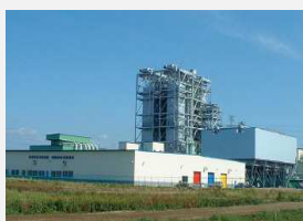
Tomakomai power plant
