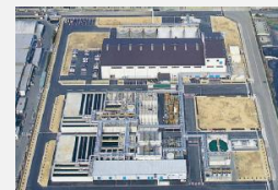
Waste liquid treatment plant
