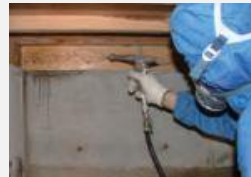
Termite control construction
