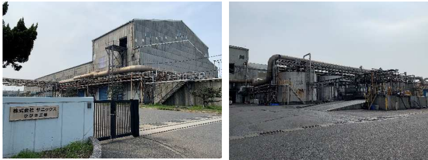
Hibiki Plant (Waste water recycle facility)
