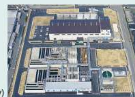
Hibiki Factory (Organic waste liquid treatment factory)
