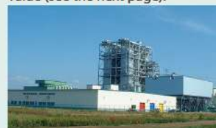
SANIX ENERGY Tomakomai Power Plant
