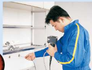
Water pipe inspection with fiber-scope
